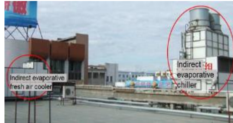
Serial water cycle system using IEC water chiller, with FCUs as terminals.
