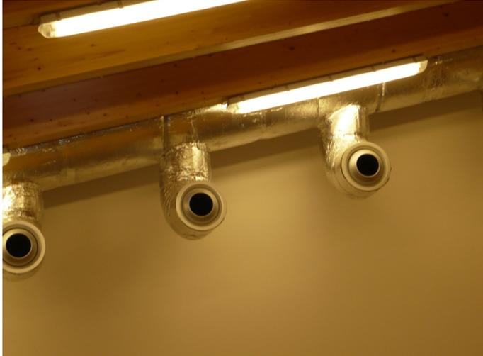
The photograph shows three ventilation ducts installed in a ceiling space. The ducts are wrapped in a reflective, silver insulation material. A fluorescent light fixture is visible above the ducts, and the ceiling structure is made of wooden beams.
