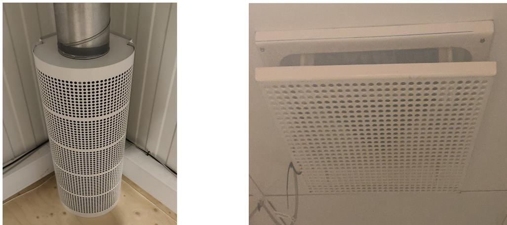
Figure 9: Pictures of the displacement ventilation diffuser (left) and exhaust (right).
