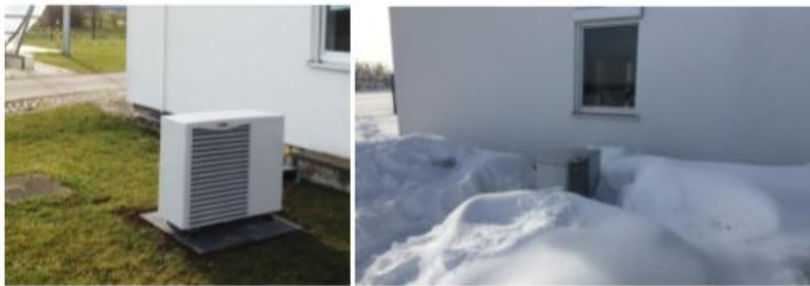
Figure 21: External installation of the Twin Houses Vaillant "aroTHERM VWL 55/2 A" air source heat pump, left in summer, right in winter.
