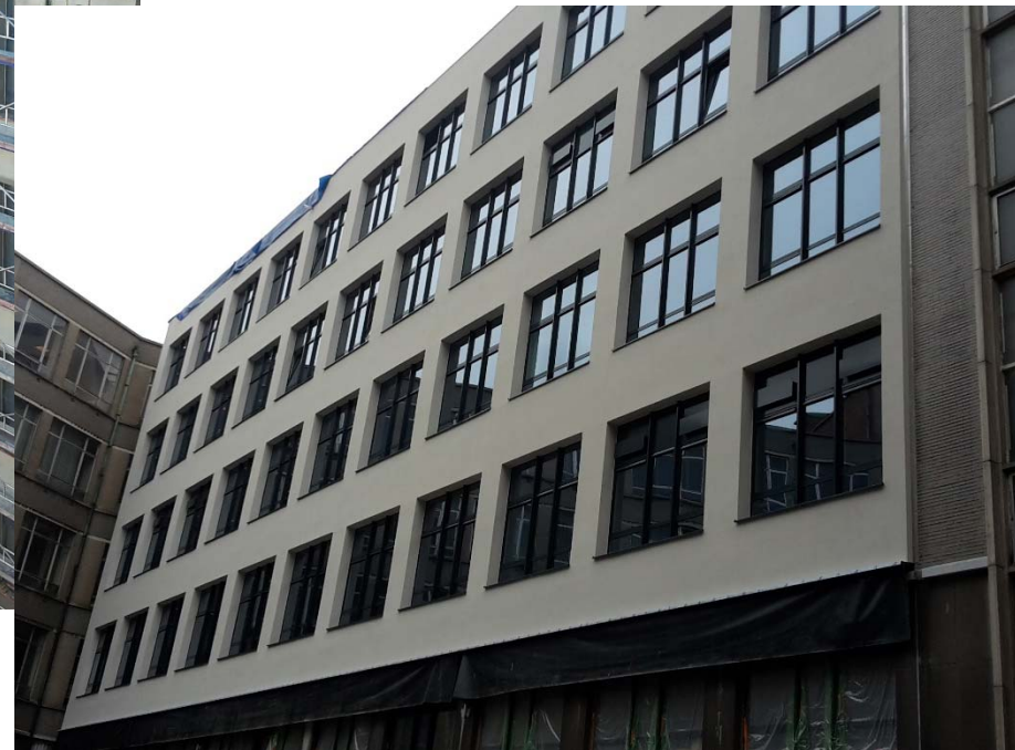
November 2016 – Finishing plaster – Block Nr 6 – Final look
