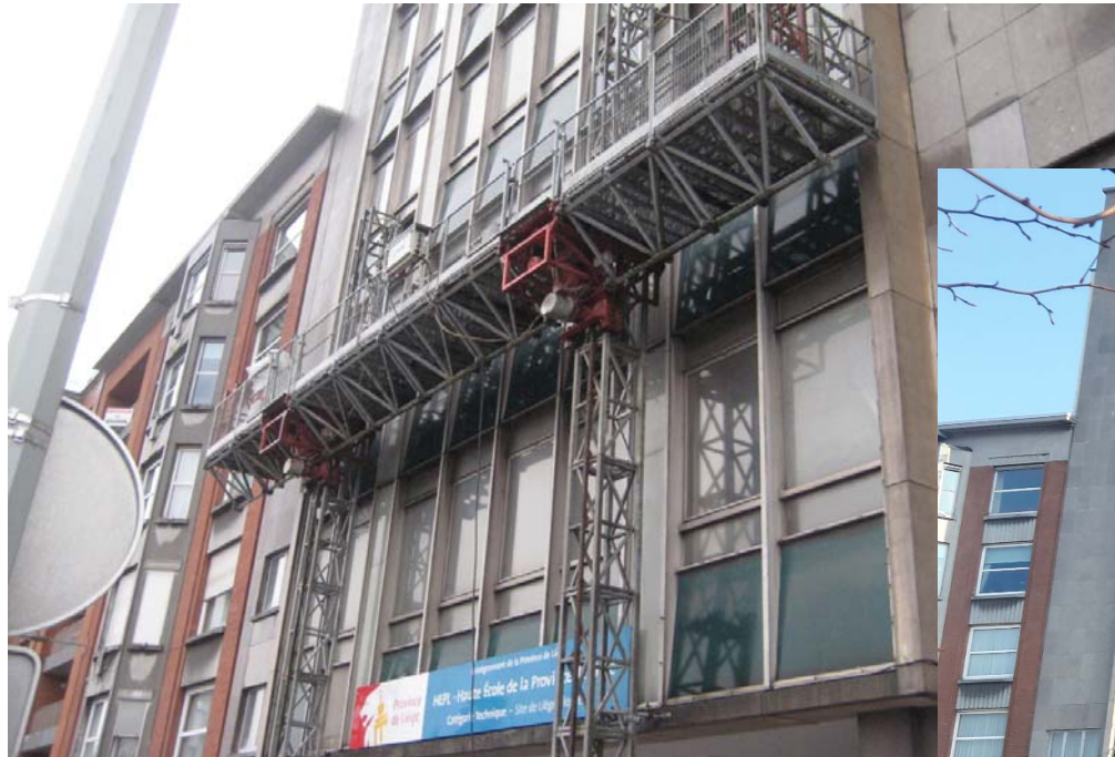
February 2016 – Installation of elevators (lifts) on site
