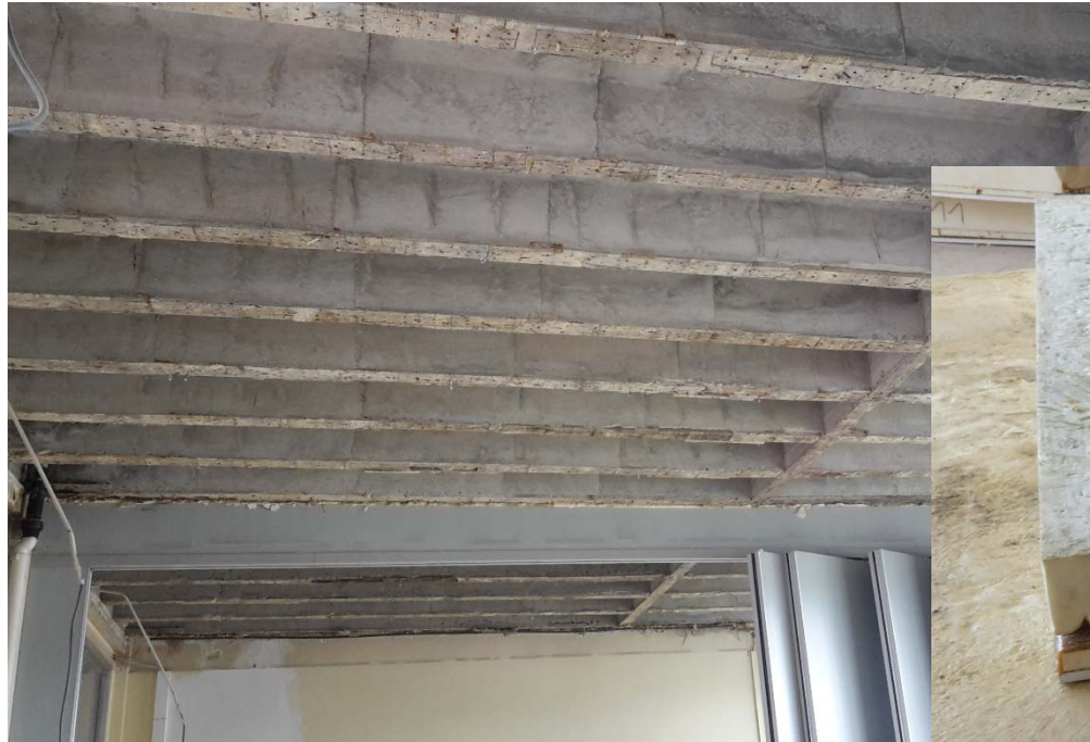
May 2016 – Dismantling of ceilings
