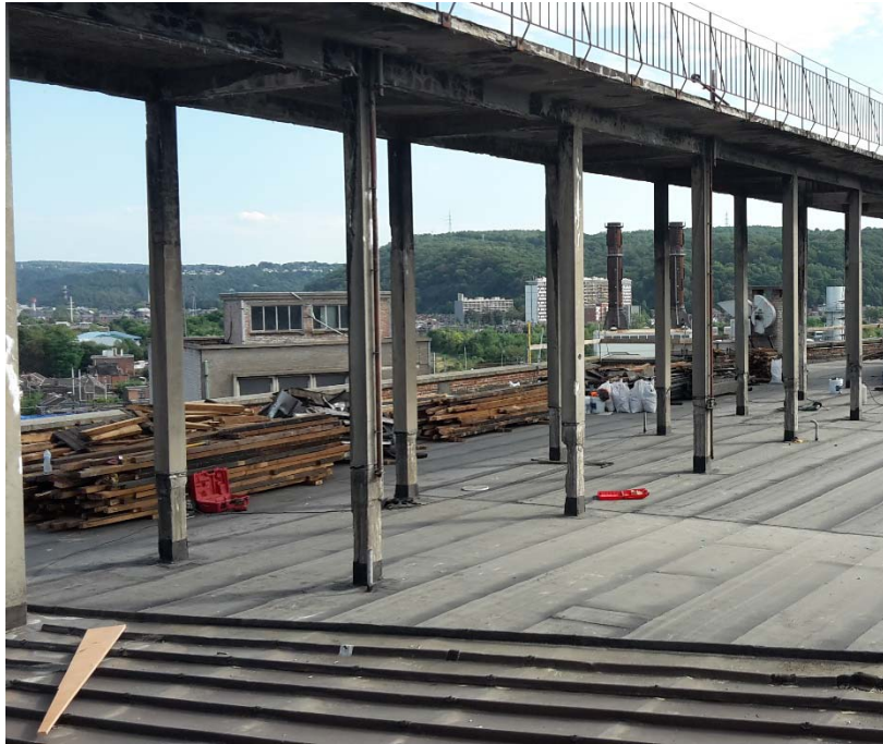
September 2016 – Works on the roof – New waterproofing
