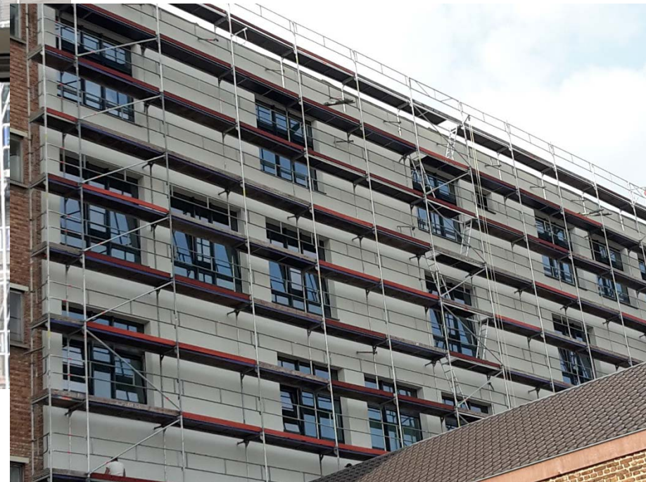
September 2016 – Finishing plaster – Block Nr 6 – Rear Facade
