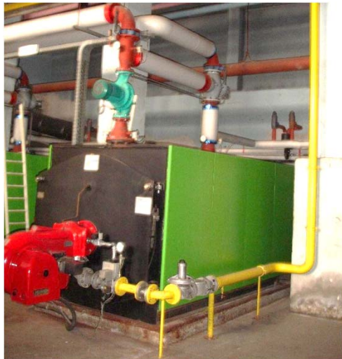
Gas boilers 3 x 2500 kW
