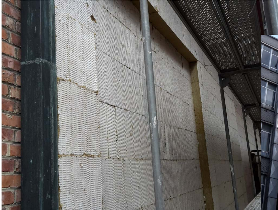
April 2016 – External insulation – Block Nr 6 – Rear Facade
