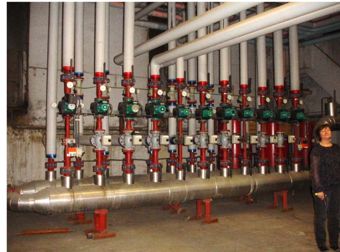
Pipe manifold 11 Heating circuits
