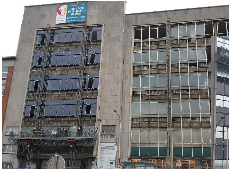
March 2016 – Rebuilding Curtain Wall A – Dismantling Curtain Wall B
