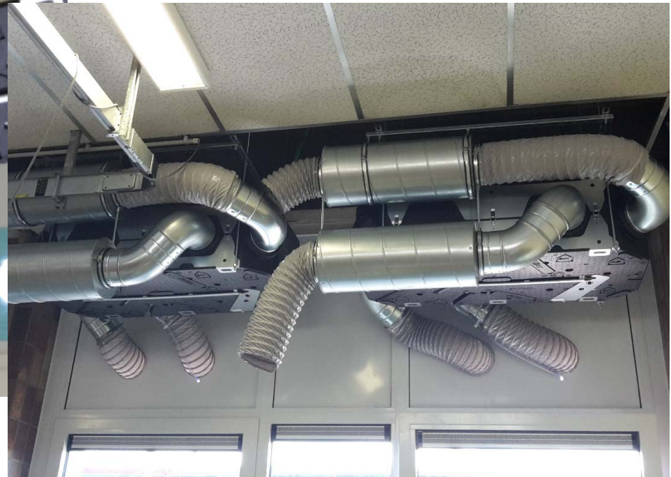
September 2016 – Air duct Block Nr 6 – Rear facade
