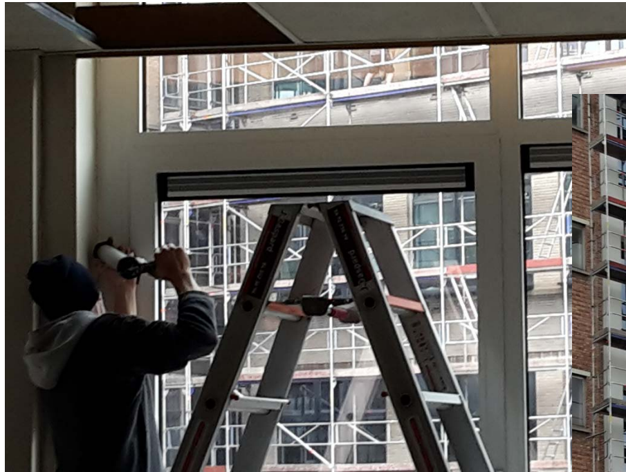
July 2016 – Internal finishing – Block Nr 1 – Facade in patio
