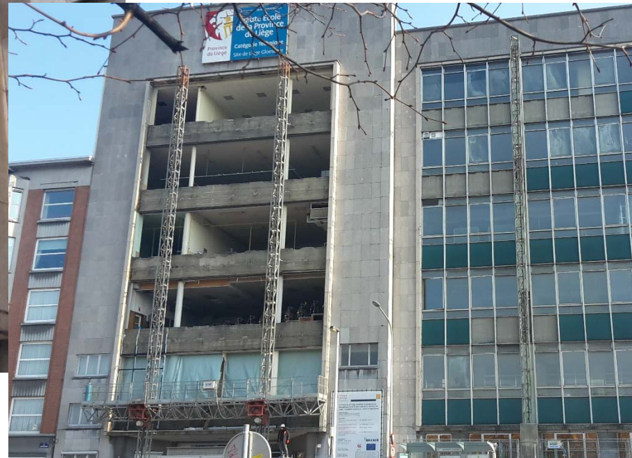
February 2016 – Dismantling Curtain Wall A
