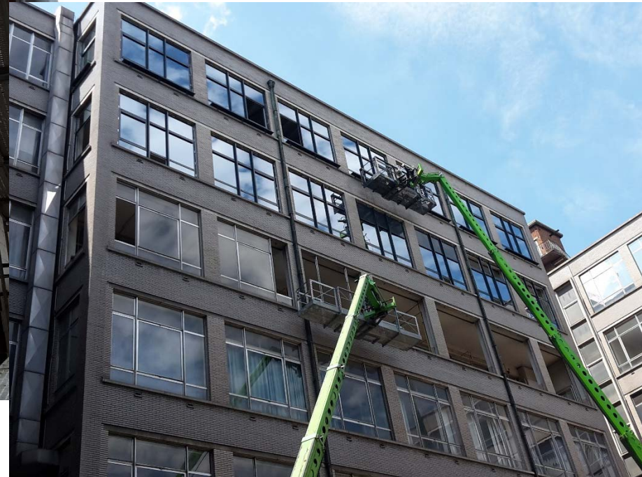
May 2016 – Replacement of windows frames – Block Nr 1 – Facade in patio
