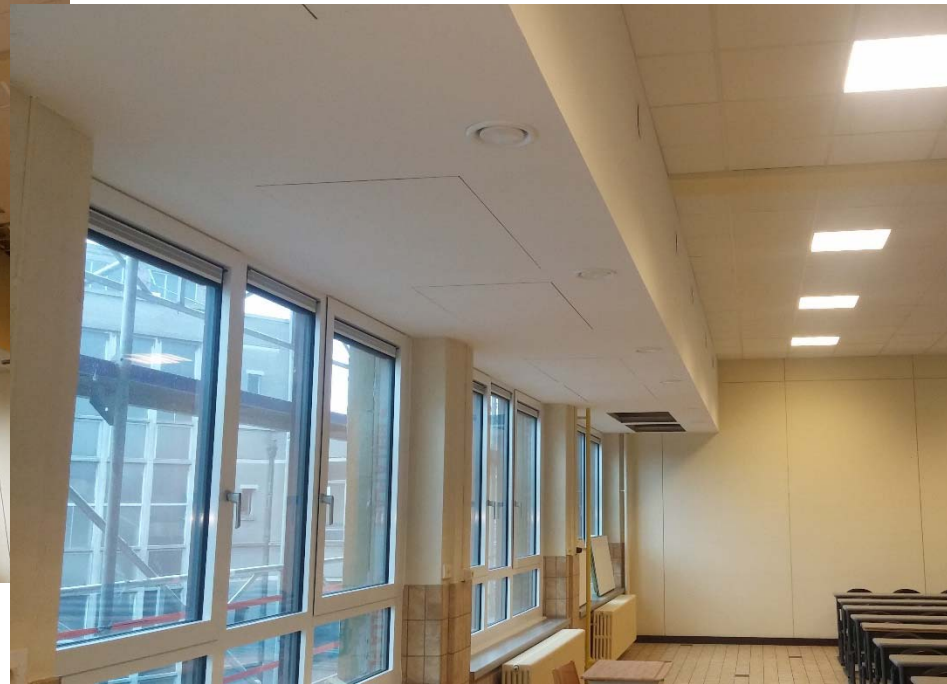
November 2016 – Smart ventilation Block Nr 1 – Final look
