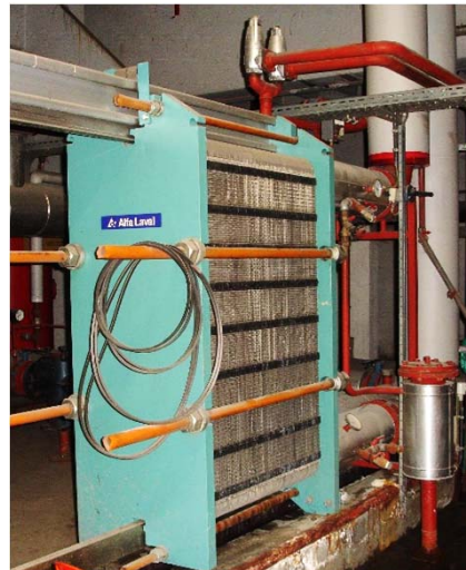
Heat exchanger 7500 kW
