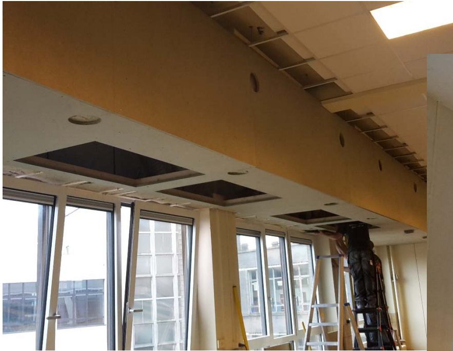
October 2016 – Smart ventilation modules Block Nr 1 – Façade in patio
