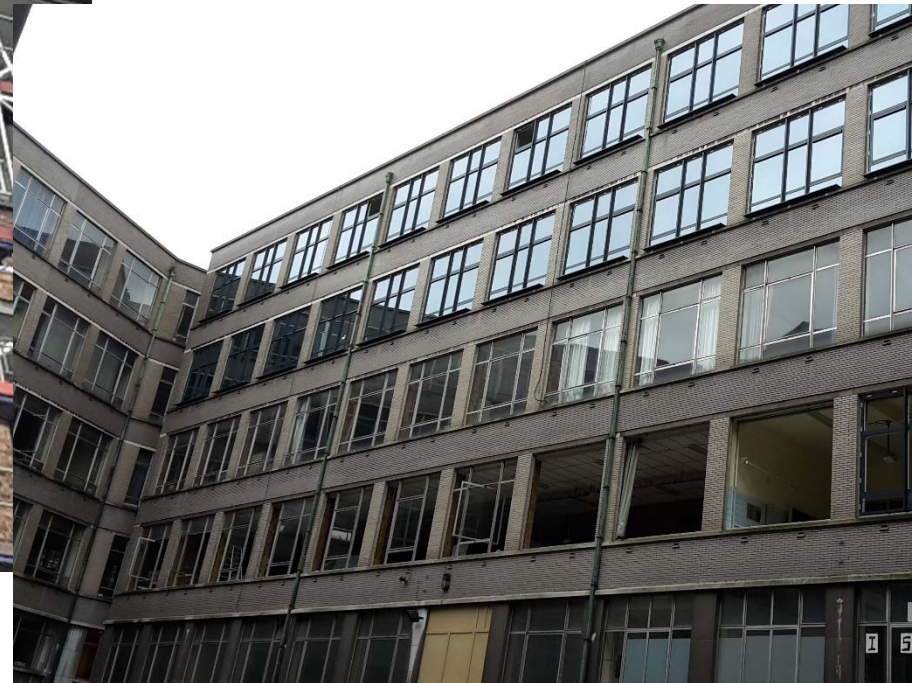
March 2016 – Replacement of windows frames – Block Nr 6 – Facade in patio
