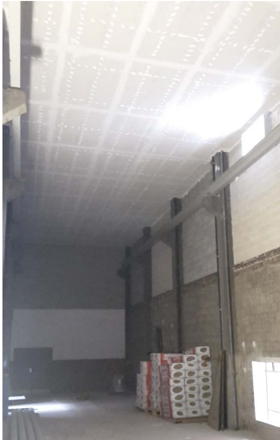
June 2016 – New heating room
