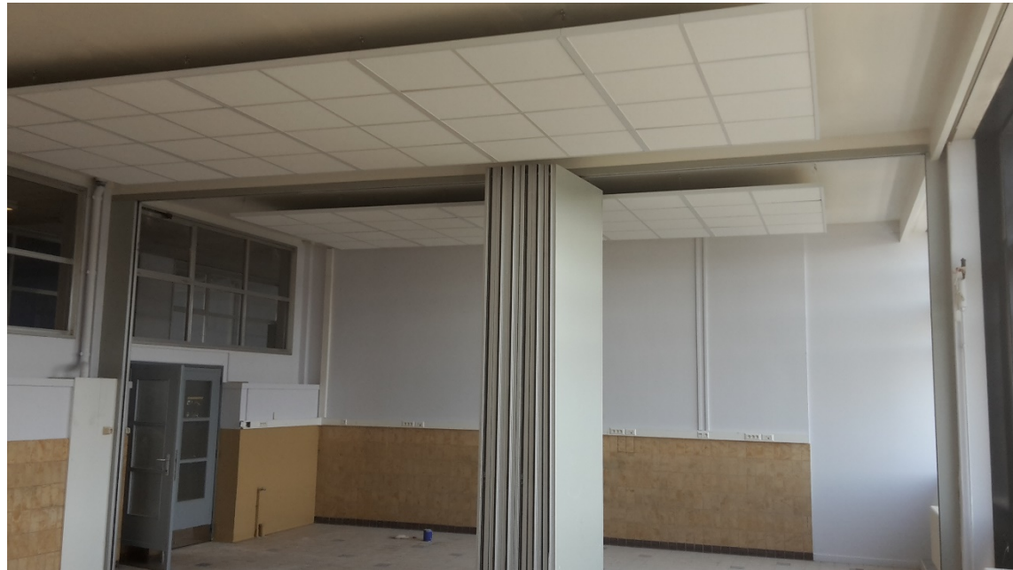
Final look of the classrooms in Level +5
