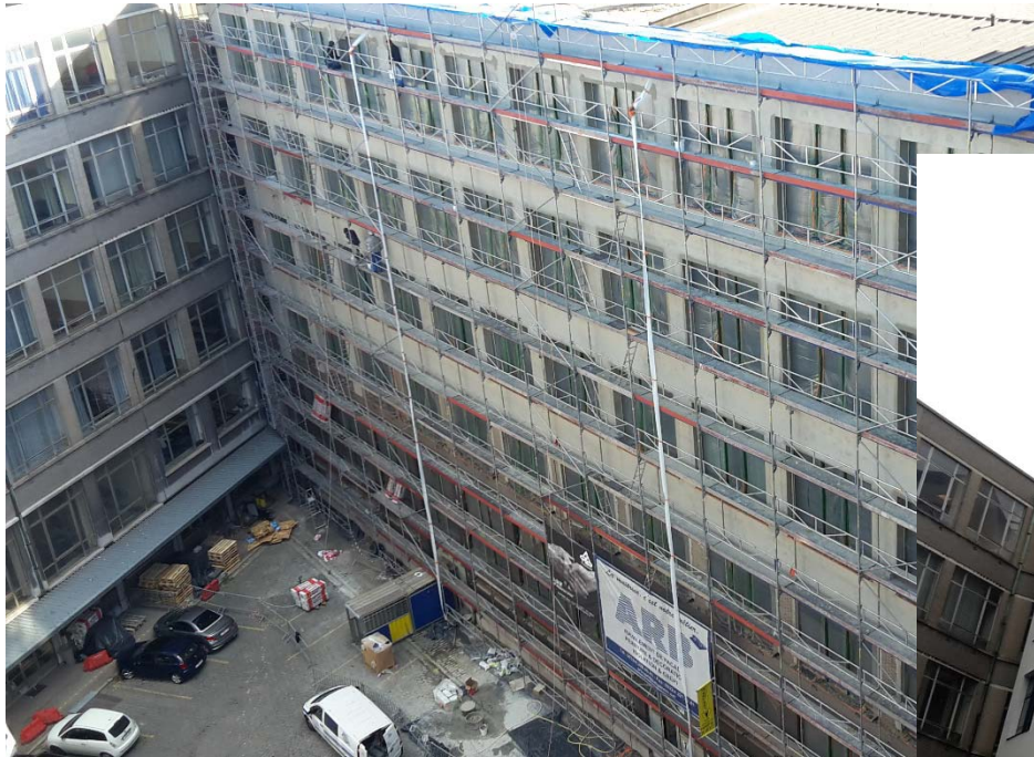
October 2016 – Insulation 14 cm rockwool – Block Nr 6 – Facade in patio
