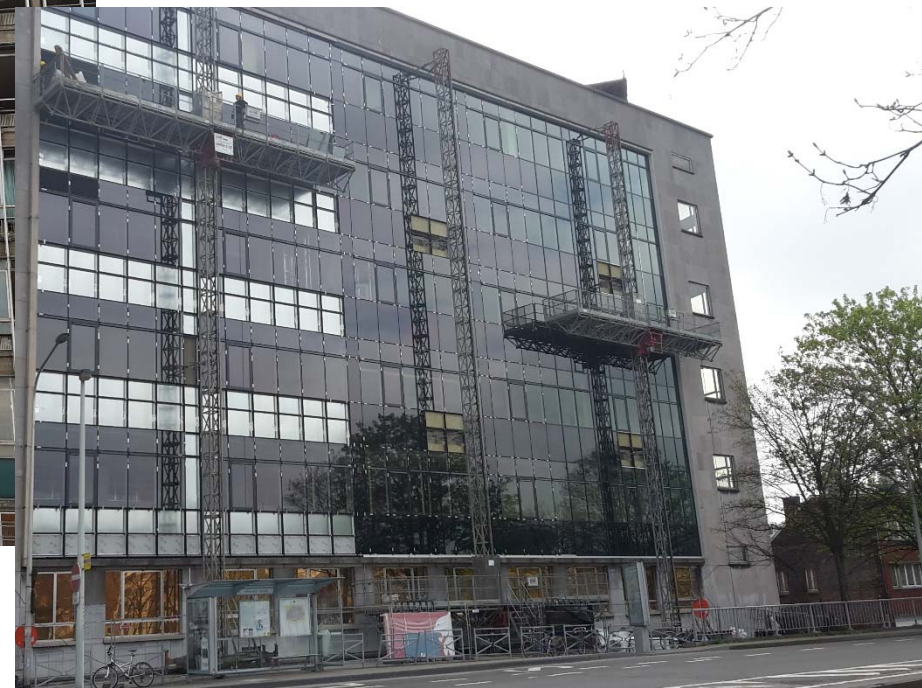
April 2016 – Rebuilding Curtain Wall B
