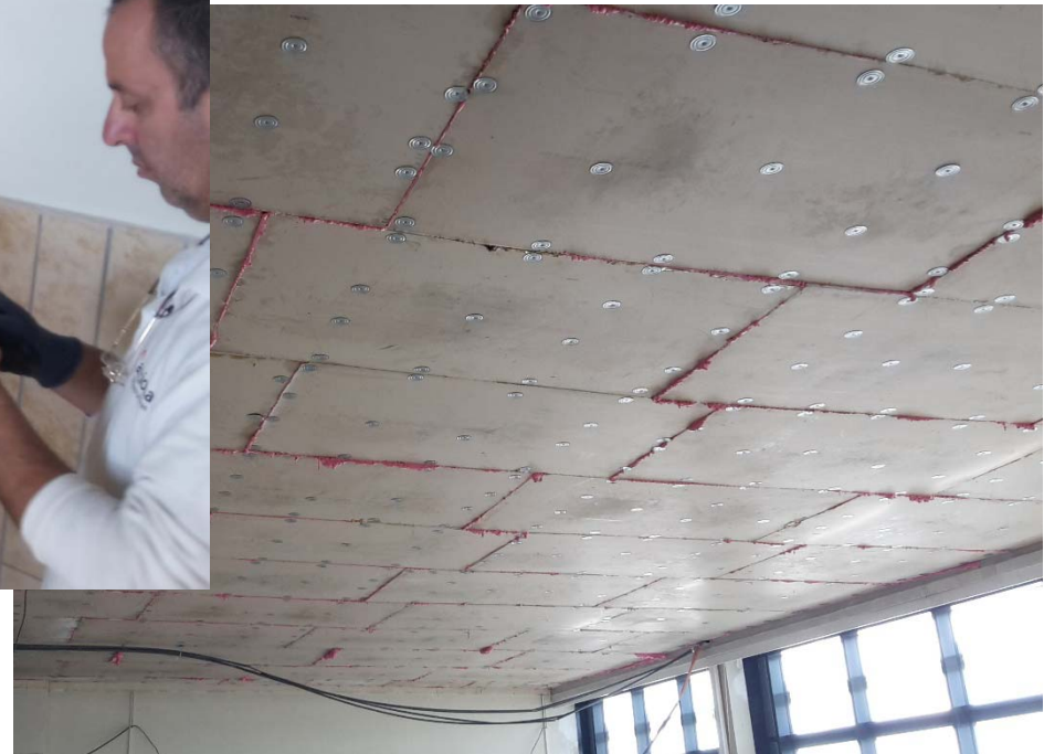
October 2016 – End of installation of Purinova's panels
