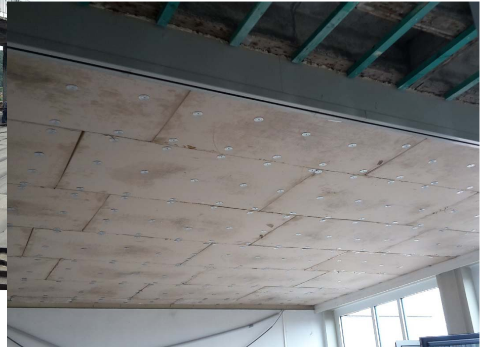
September 2016 – Installation works of Purinova's panels
