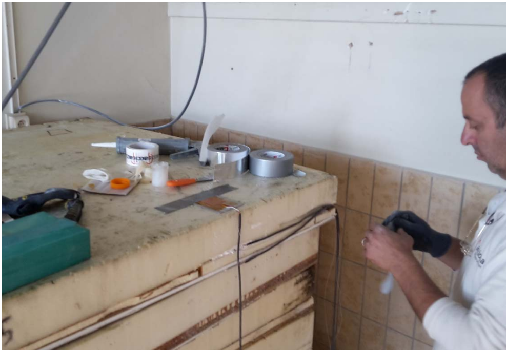
October 2016 – Acciona installs sensors into Purinova's panels – Post-monitoring
