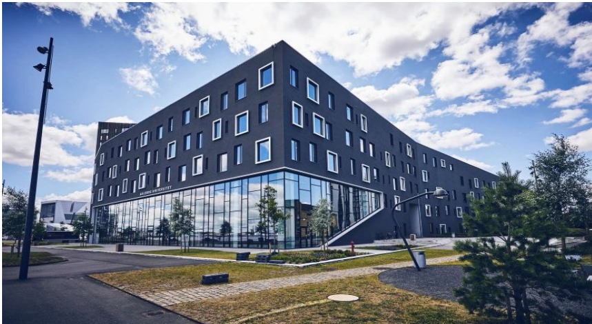
Office (university) building: 20 694 m 2 , 4 floors, 4450 people max, suffer from overheating, Denmark, Desiccant Evaporative Cooling System (Source: Aalborg University)
